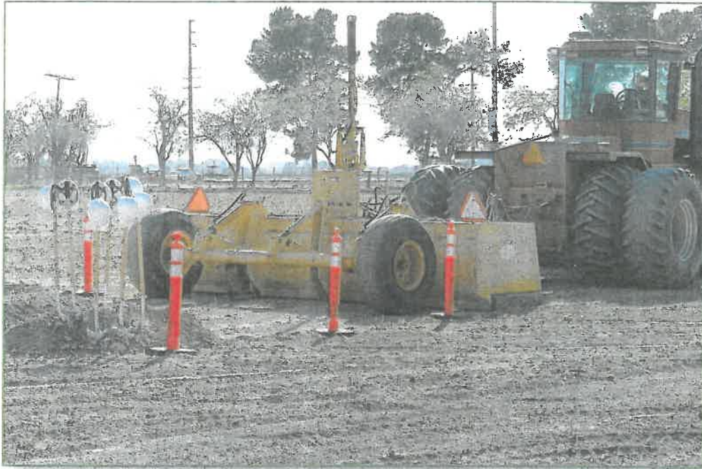
Freedom Park Baseball Field Construction
