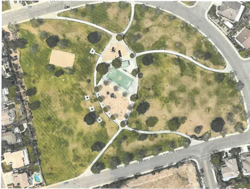
Figure B.1.3 General Overview of Lokker Park
