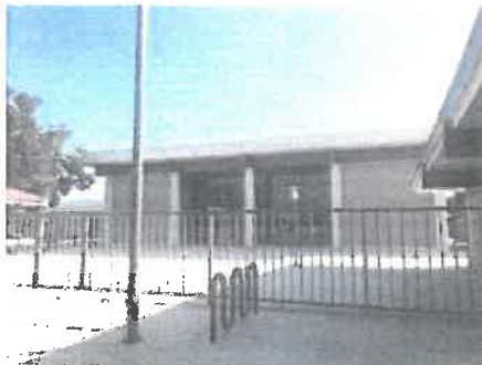
Photograph 2. View of the Community Center Building, facing north.
